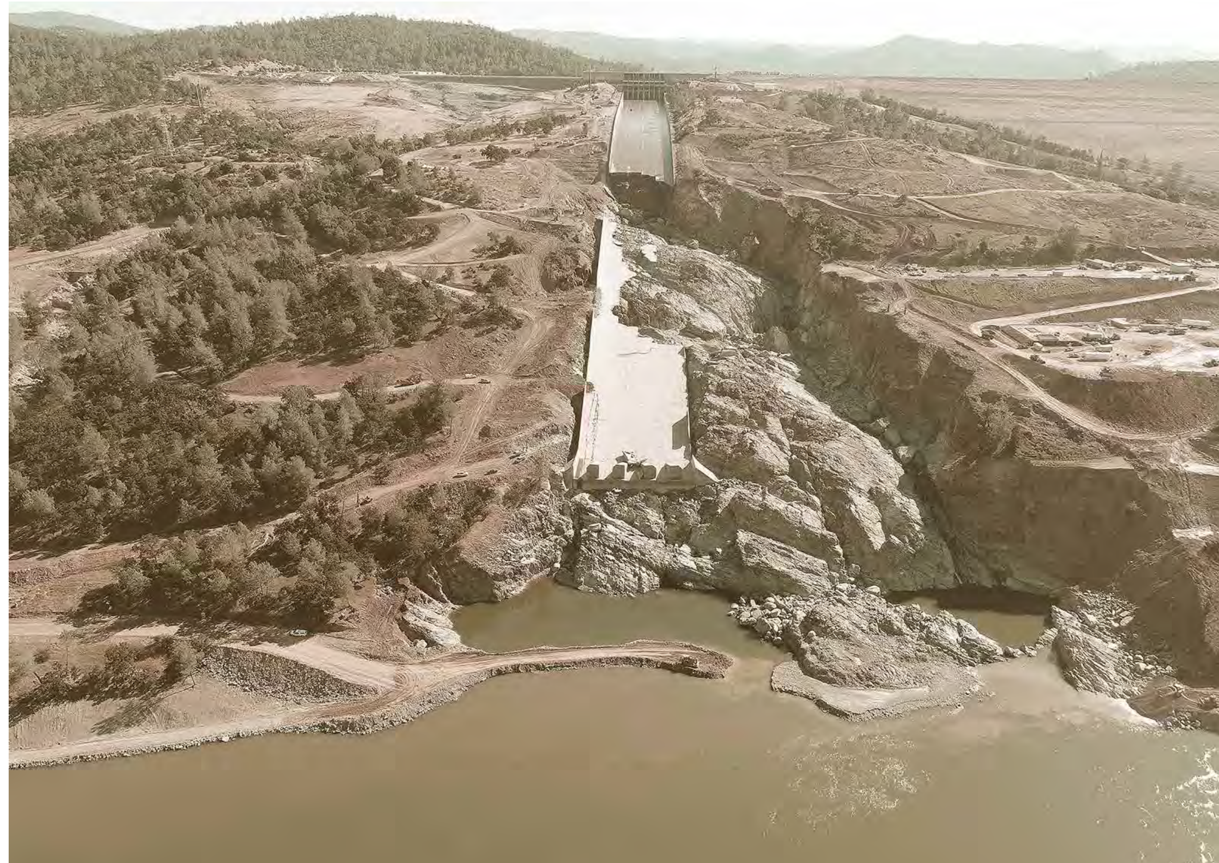
↑ Excessive rainfall in California in 2017 resulted in the use of the emergency spillway at Oroville Dam for the first time in 50 years.
